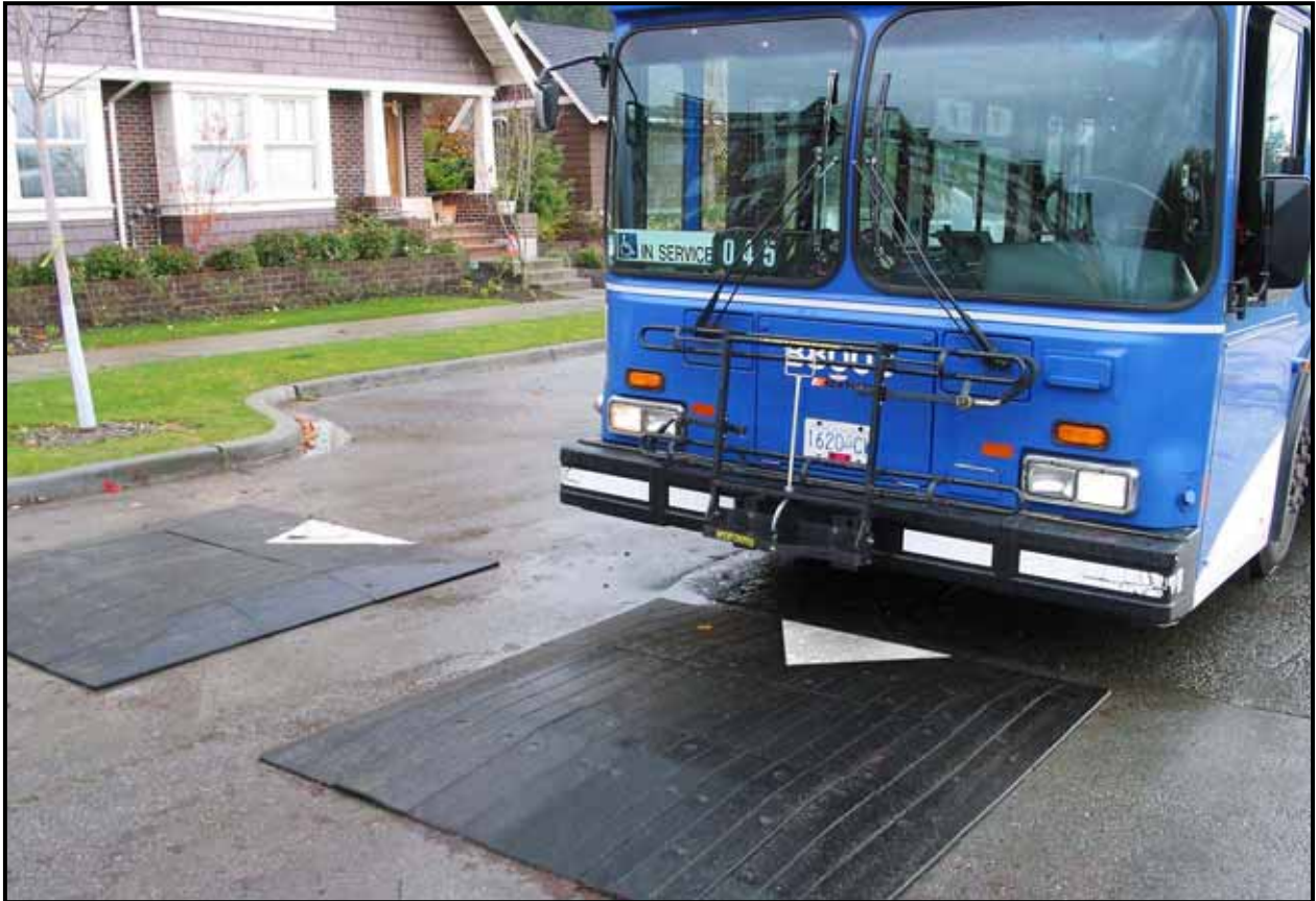
Figure 4.2 Speed Cushions with Transit Bus
